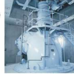
Dewatering pump with adjustable vane (Size: 2400mm, Driver: 1103kW)
