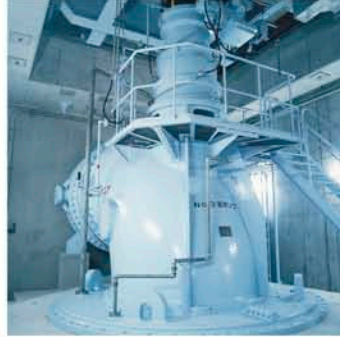
Dewatering pump with adjustable vane (Size:2400mm, Driver:1103kW)
